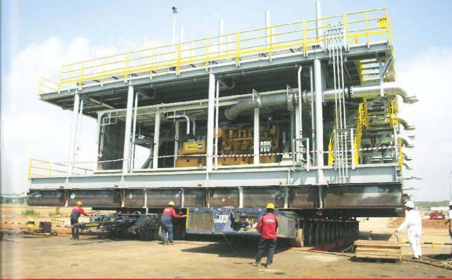
Pipe Deck Aft Module, Dim. 24.7m x 19.1m x 5.5m (413 Tons). Land transport from fabrication yard, loaded onto barge and transported by sea to Singapore.
